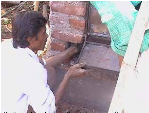
Bottom door being fixed for ease of move-
